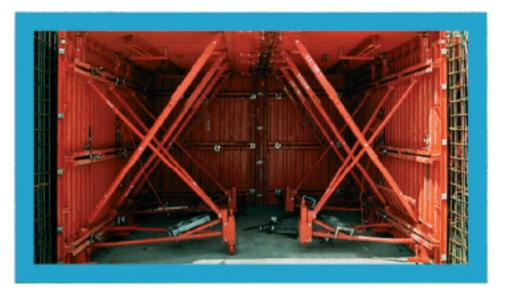
Although this technique was invented 50 years ago, of late, this method of construction has become popular and gained momentum in building construction with the integration of modern technology. The use of hydraulically operated jacks and wheels to the pre-fabricated structural steel shutter plates made it easy for the Formwork to move in and out of the position and adjust the final height of the building block to achieve the desired size.
